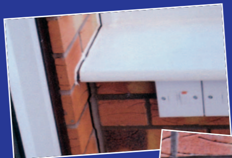
This photograph shows 'lateral cracks' in the mortar beds of a recently built conservatory, displacement of this type can be readily caused by incorrect foundation design, rebuilding would be required.
